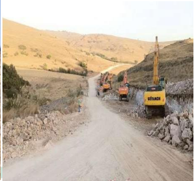
Excavation in rock for ROW construction 2
