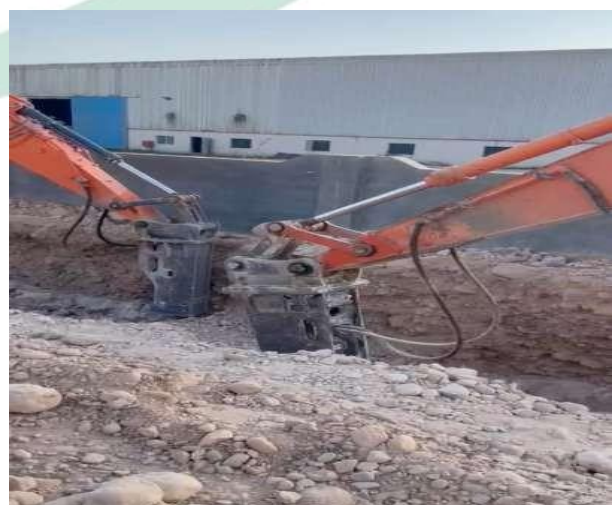
Rock Breaking in Progress RAYSUT
