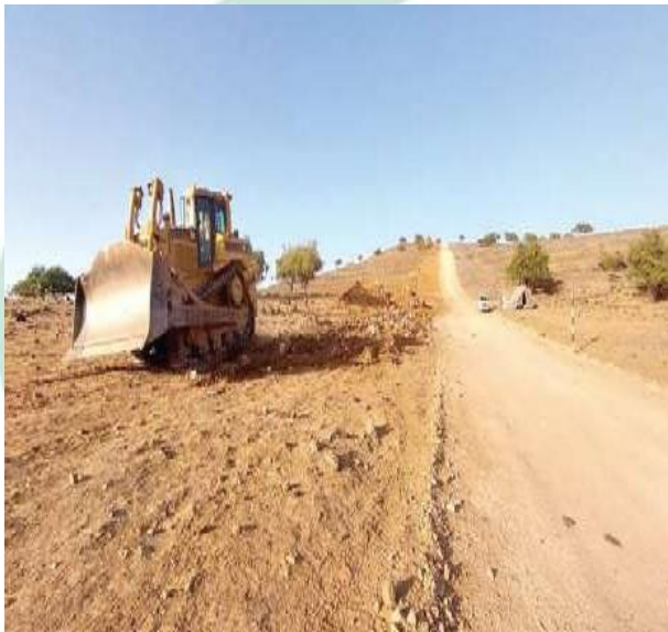
Dozing in Progress for ROW construction
