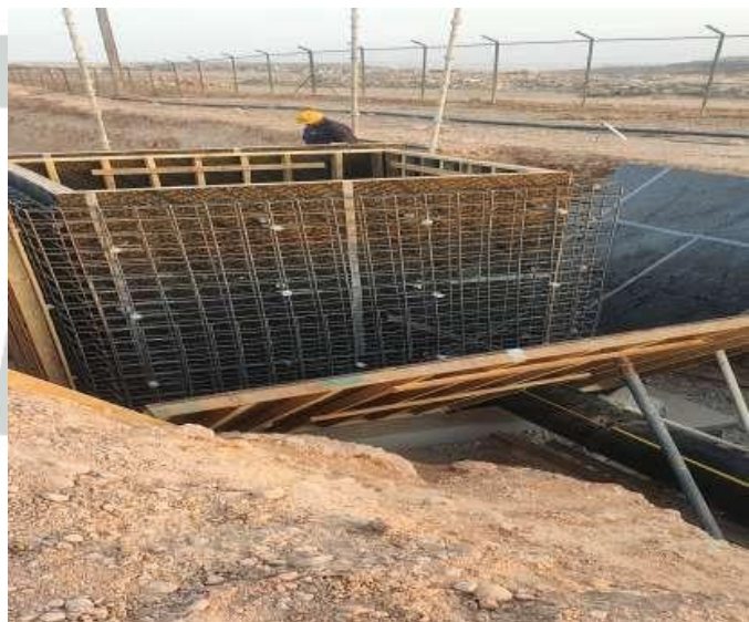
Valve pit construction in progress
