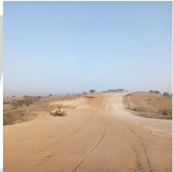
Grading and compaction for ROW construction
