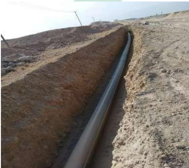
20" HDPE Pipe laying
