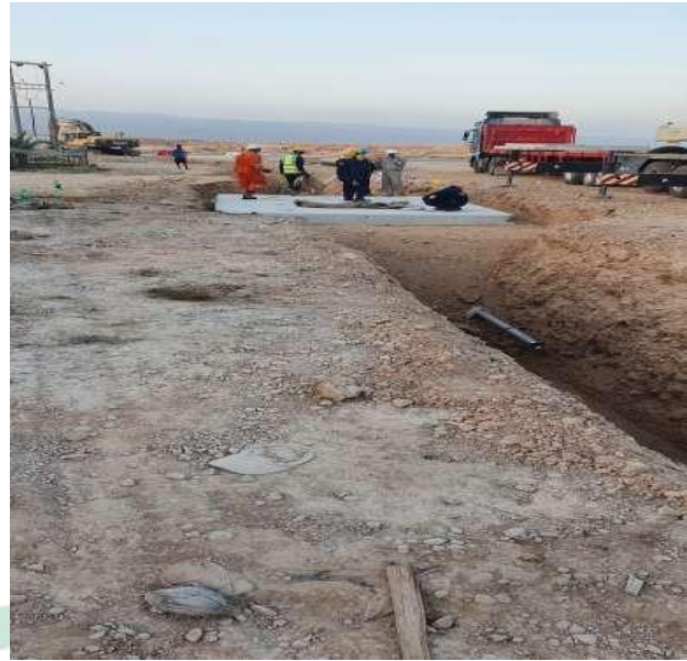
Precast Slab Installation For Road Crossing
