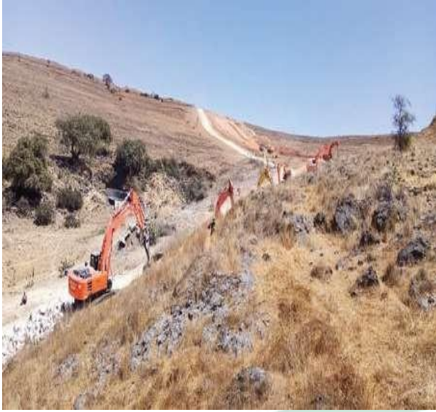
Excavation in rock for ROW construction1
