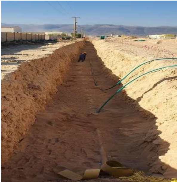
Foc Duct Installation Works Raysut
